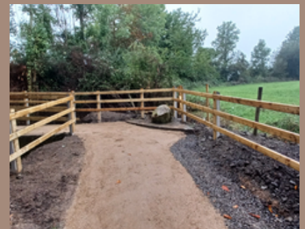
After Upgrade Works
